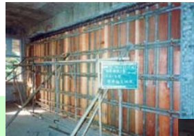
Replace brick wall to infill RC wall
