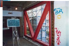
Retrofitting by steel brace
