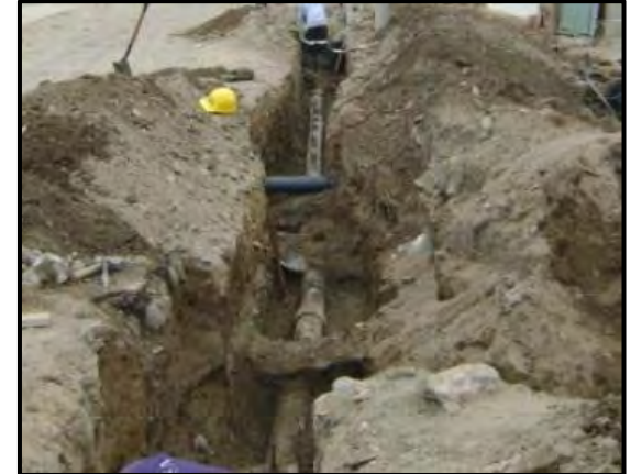
Replacement of AC pipe for PVC pipe
