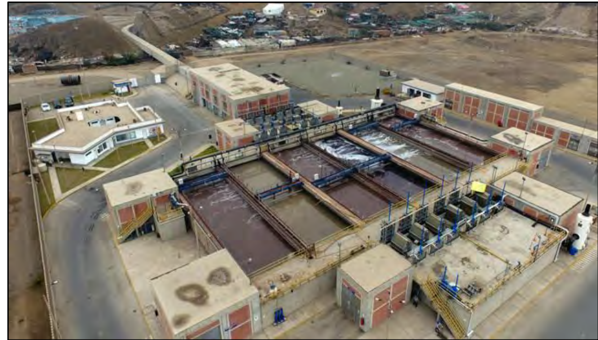
Wastewater Treatment La Chira Plant
