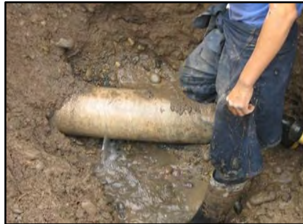
Leak AC pipe
