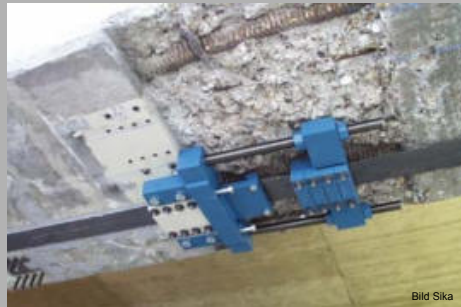
prestressed CFK- elements
