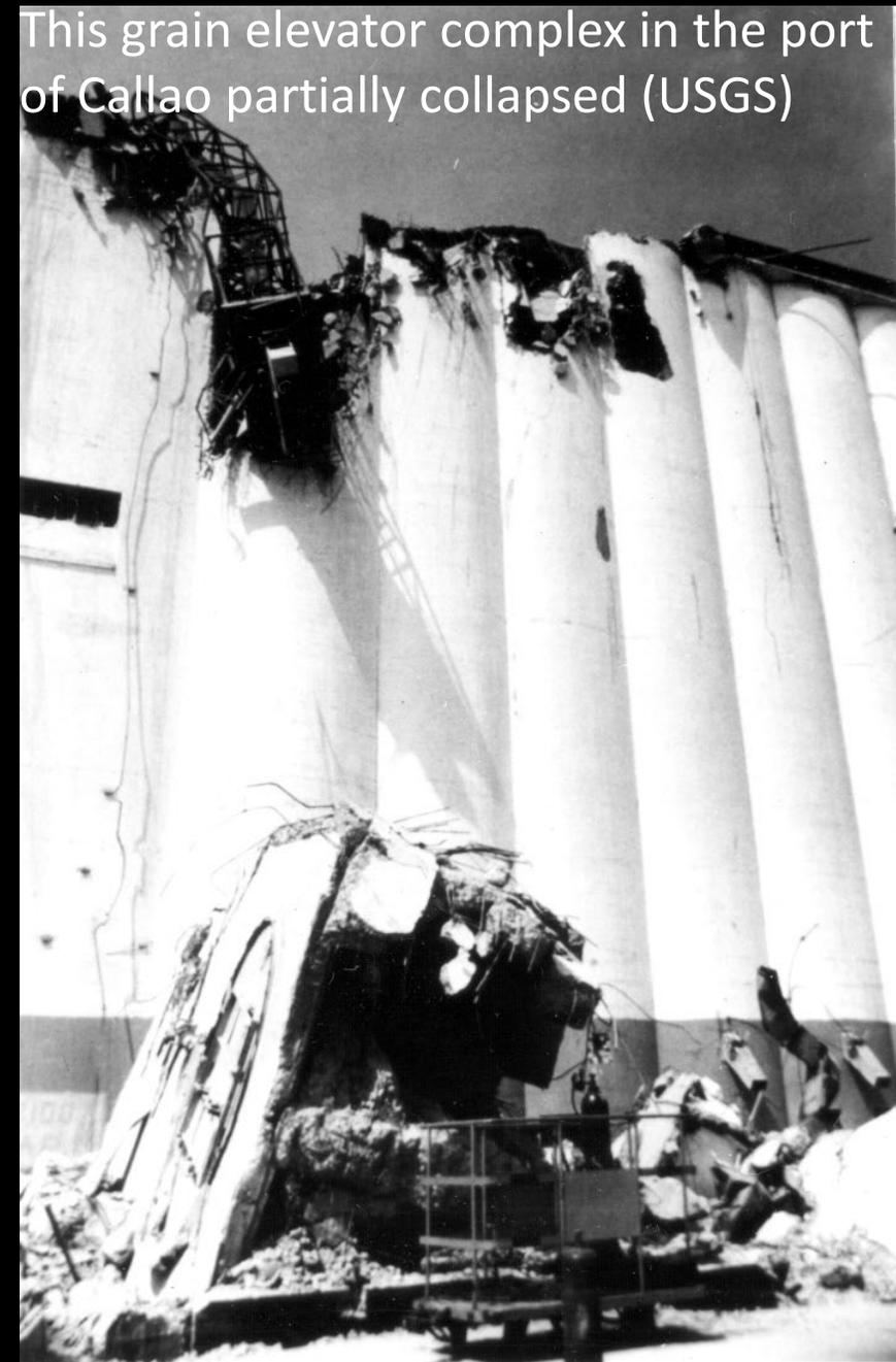
**This grain elevator complex in the port of Callao partially collapsed (USGS)**
