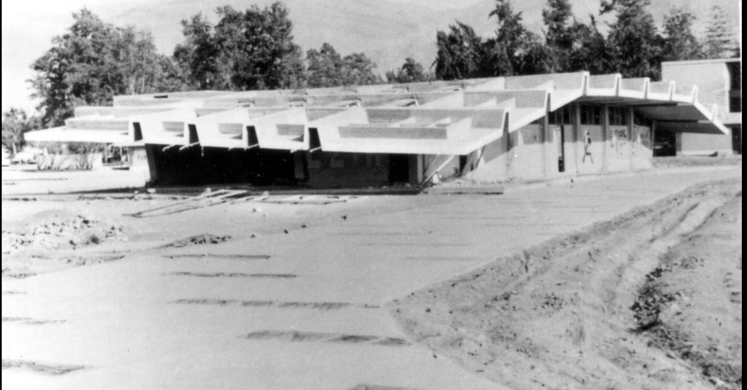
Example of the extensive damage in La Molina District. This classroom and a laboratory building at the Agrarian University partially collapsed, 1974 (USGS)
