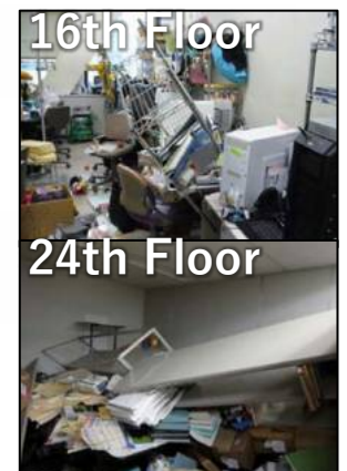
Overturning of Shelves Kubo et al., 2014
